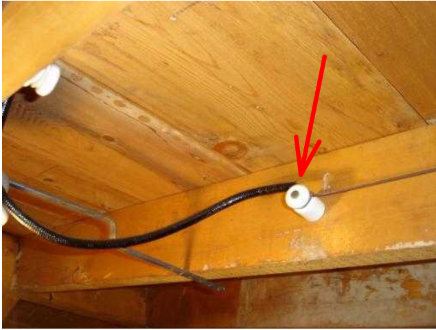
Knob and tube wiring
